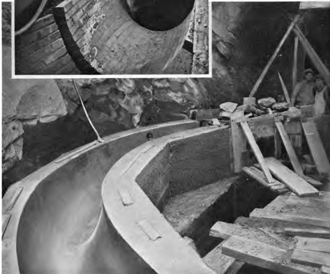
CONCRETE SEWER BACK OF ELECTRIC DUCT MANHOLE — BROADWAY AND 58TH STREET
